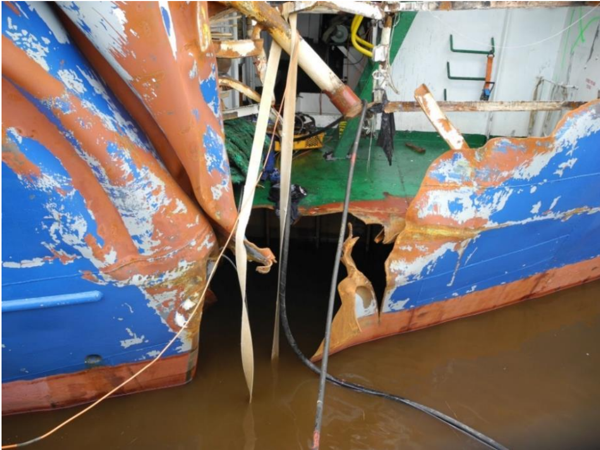
Figure 4: Breach at the waterline 5
