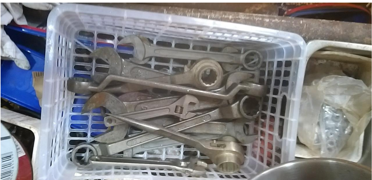
Non-sparking tools stored in the compressor room
