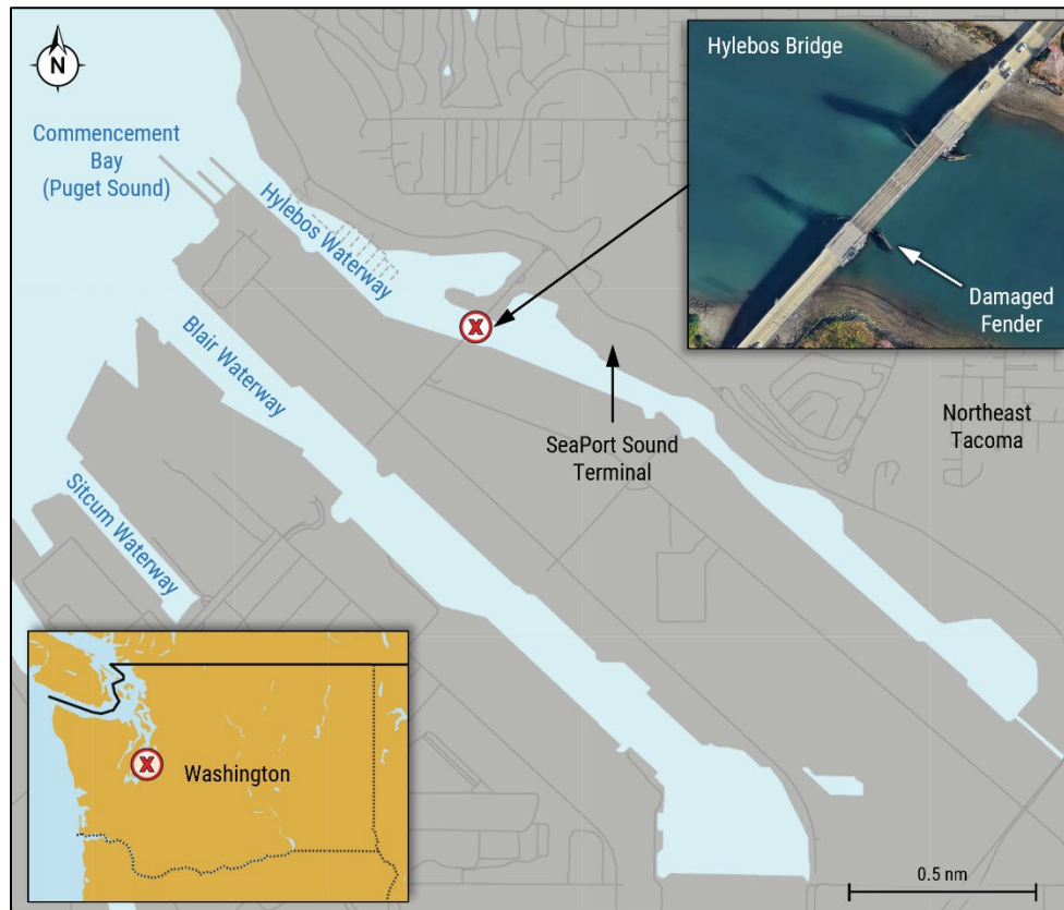
Figure 2. Area where the Olympic Scout contacted the Hylebos Bridge fender, as indicated by a circled X. (Background sources: Google Maps [maps], Google Earth [bridge image])
