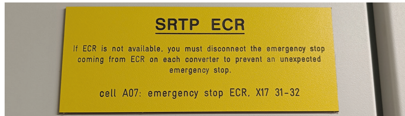
FIGURE 41. SRtP instruction to disconnect the emergency stop signal from the ECR (if lost) to each propulsion converter to avoid an unexpected loss of propulsion
