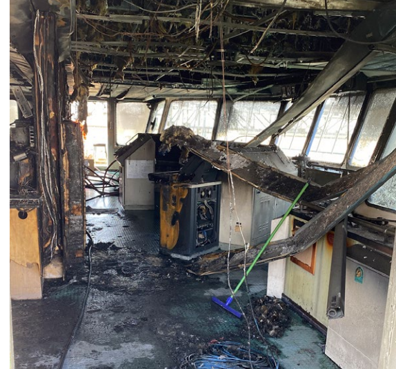
The damage to the bridge. SOURCE: COAST GUARD
