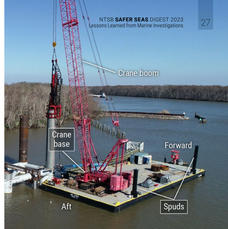
Crane barge Mr. Dawg in operation.
