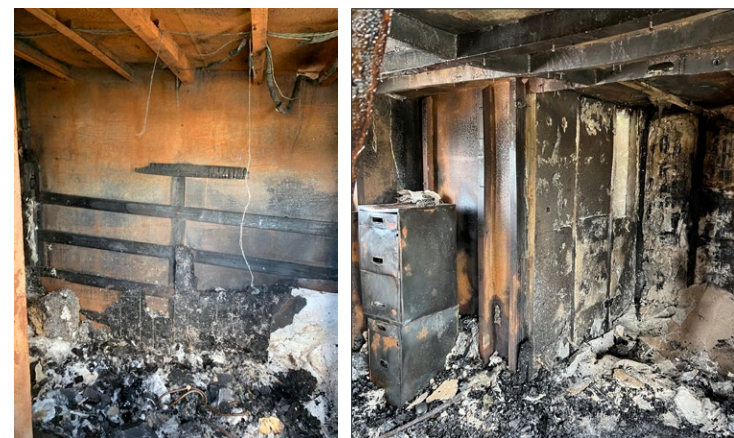
Left to right: Charred wooden framing attached to steel bulkhead and pilot's stateroom adjacent to the starboard stack where the fire started. SOURCE: NTSB
