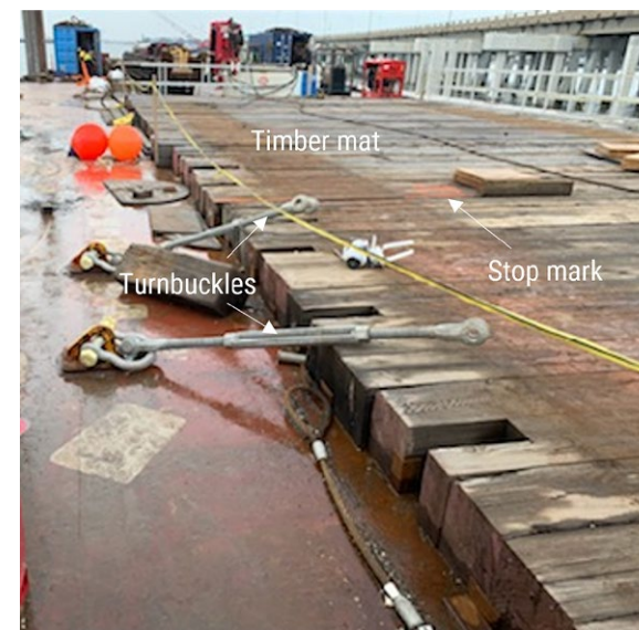
Location of turnbuckles near timber mat and stop mark painted orange on the mat.
