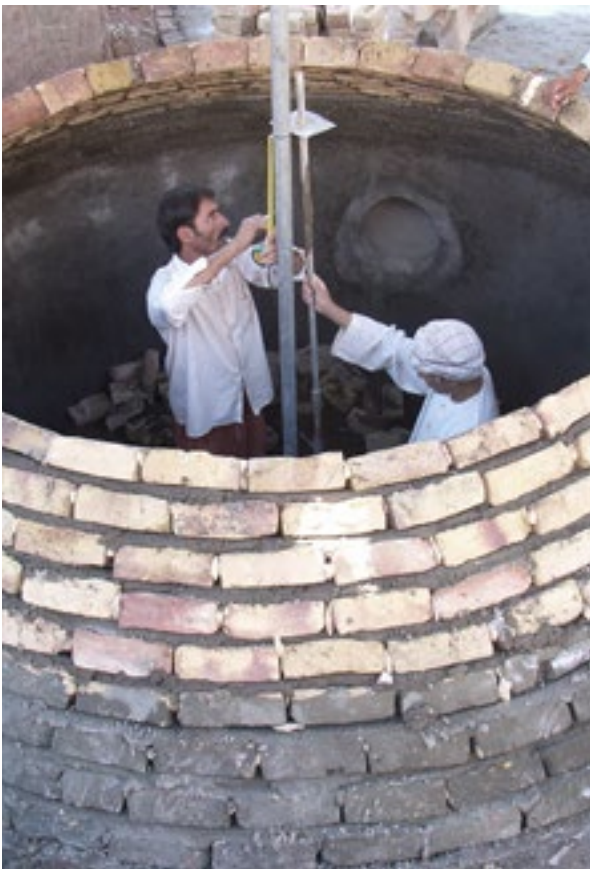
Figure 10: Small-scale digester dome construction in Afghanistan.
