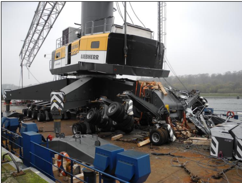
Figure 14: Buckled machinery housing, destroyed running gear 22 The left rear supporting pad had torn away from the support base.
