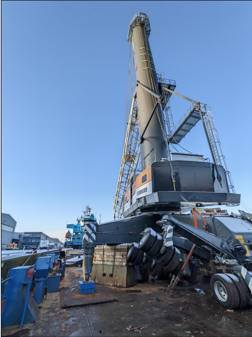
Figure 18: Secured crane. Photograph taken on 9 December 2022 26
