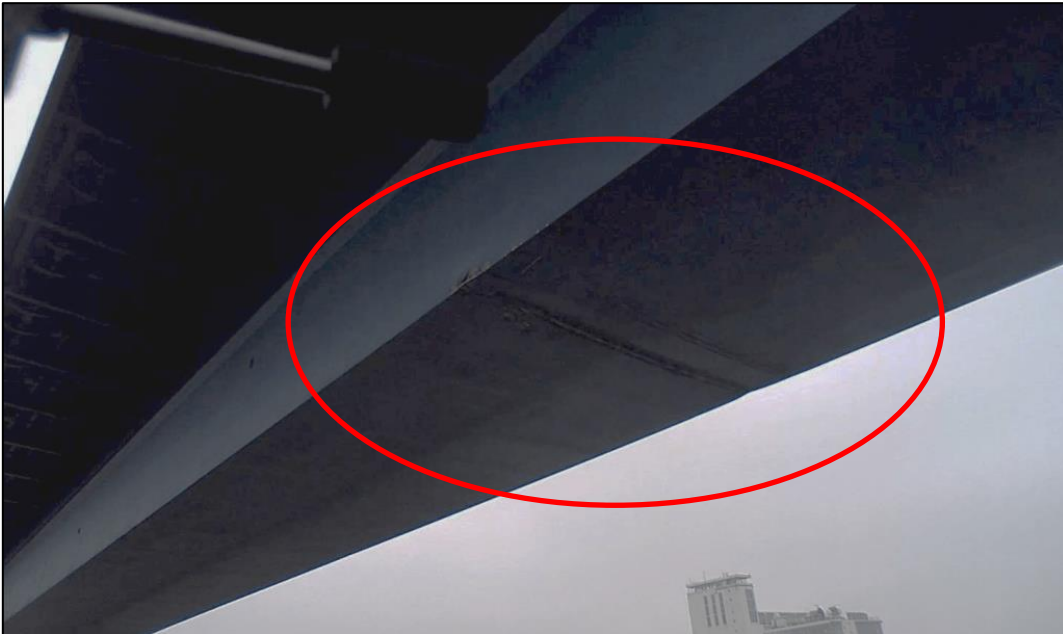
Figure 21: Prinz-Heinrich-Brücke bridge (western Holtenau high bridge) 29
