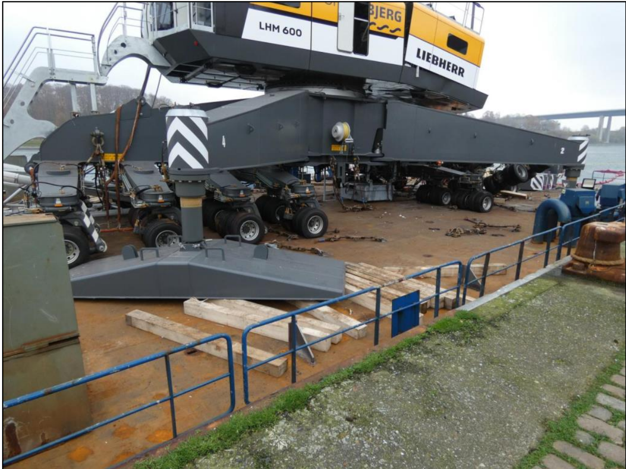
Figure 15: View of the left-hand side of the crane 23 The steel support base was broken. The forward left supporting pad no longer stood on the wooden substructure. The machinery housing was buckled.
