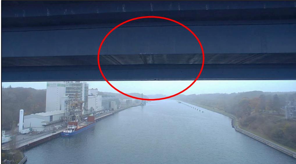
Figure 19: Olympiabrücke bridge (eastern Holtenau high bridge) 27
