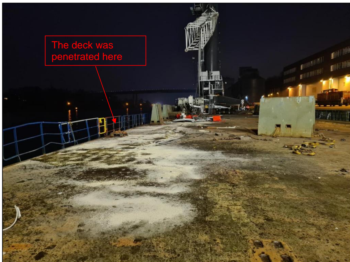
Figure 12: Cargo deck of the MERI 20 View to aft. Inter alia , the oil binding agent on the upper deck and the buckled railing on the starboard side (front left in the photograph) can be seen.
