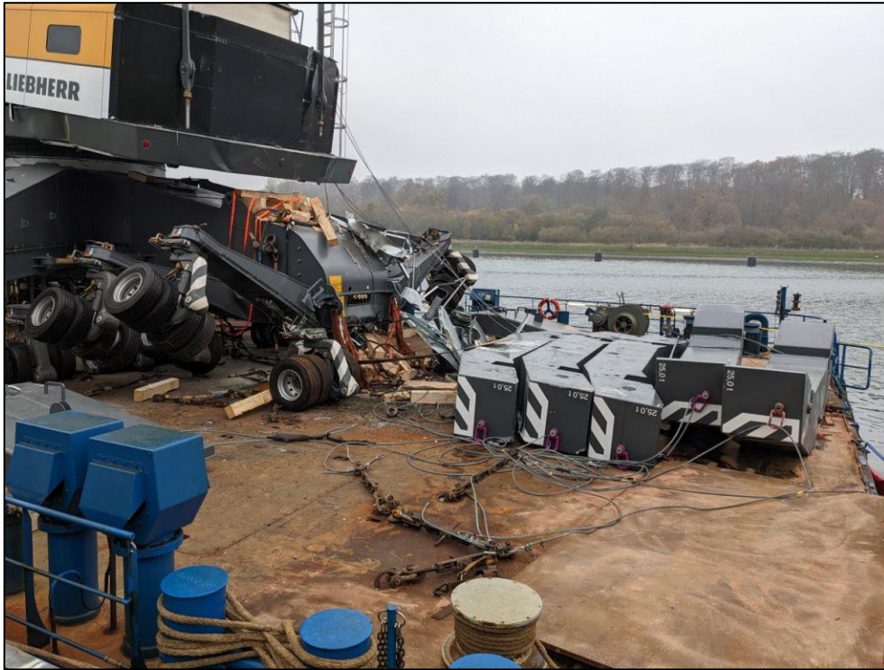
Figure 13: Fallen counterweights 21 Part of the railing is missing from the stern, which fell into the canal with three counterweights.
