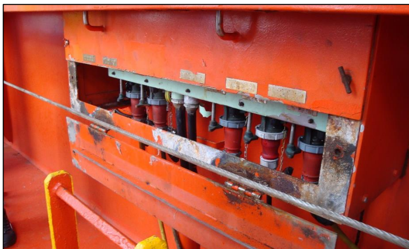
Figure 4: Terminal/switch box (lower access panel open)
