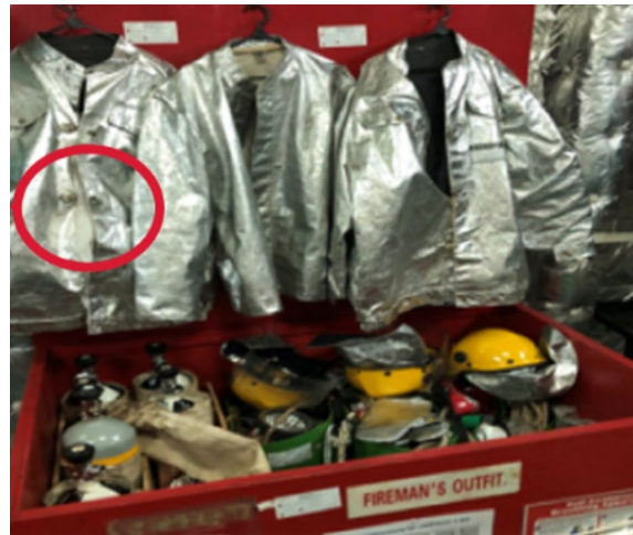
Figure 1: Suits with unprotected metal buttons do not provide the necessary thermal insulation.
