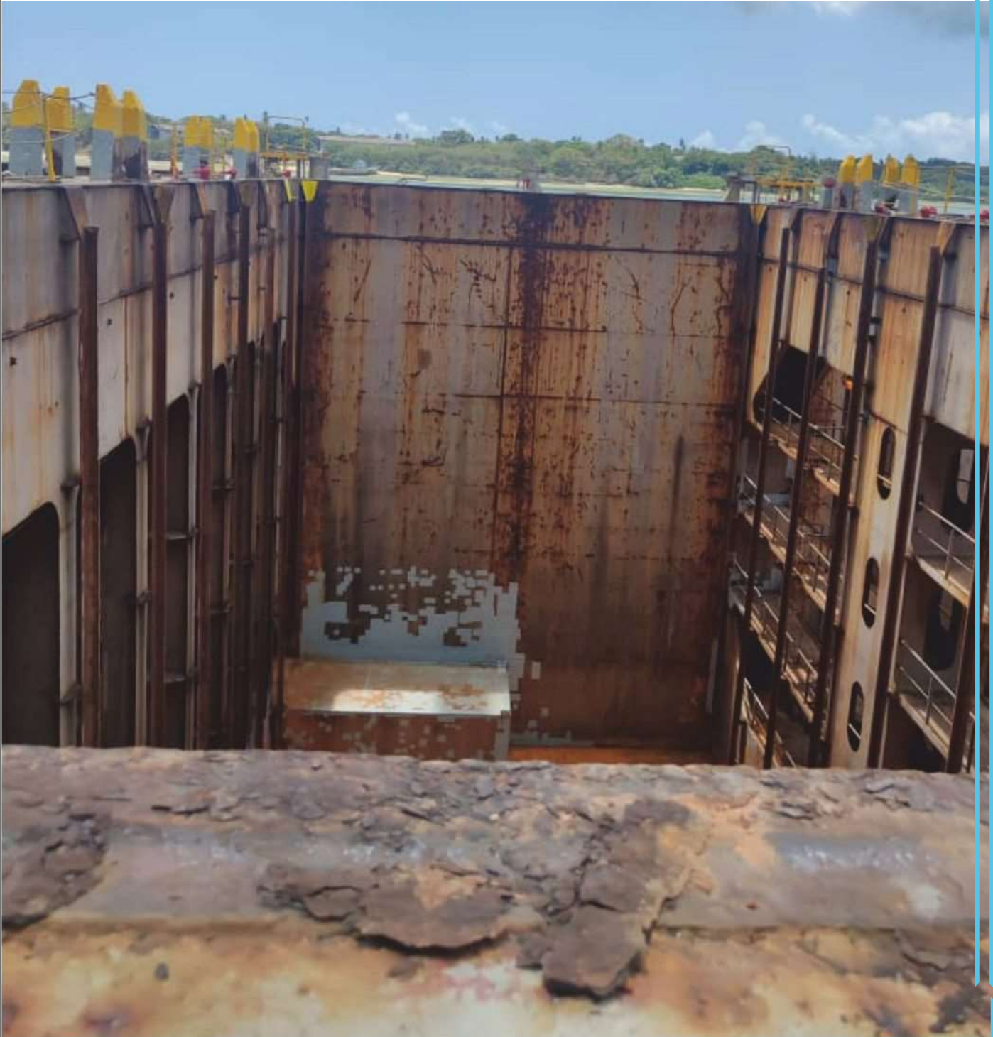
Cargo hold corroded
