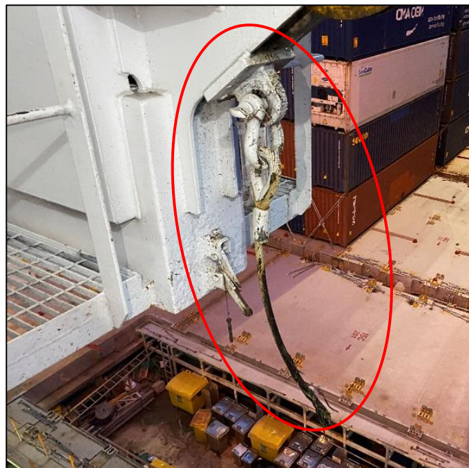
Figure 5: The fixed end of the monorail crane's parted wire (port side)
