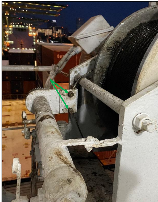
Figure 11: The additional bolts (green arrows) that were found installed
