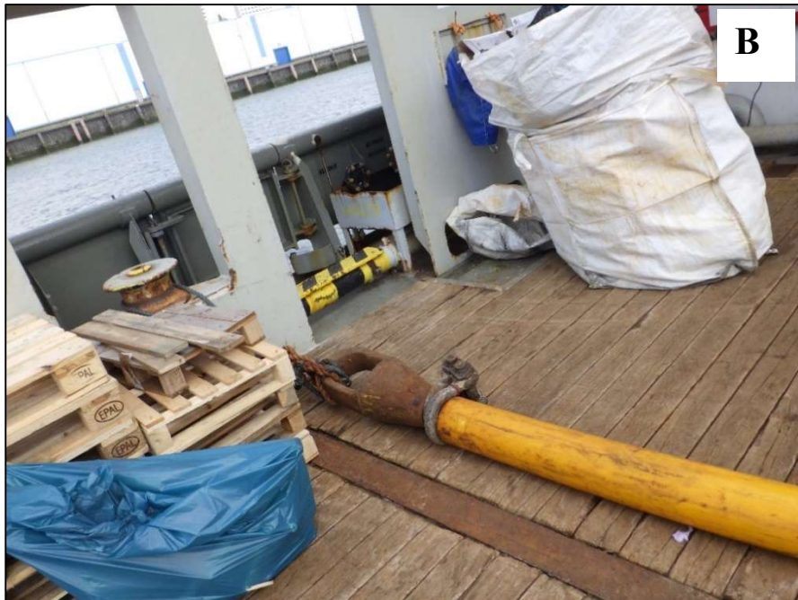
Figures 24 A and B: A showing the steel towing wire on the winch and B, the end of the same steel towing wire. The Dyneema towing line was attached to this towing wire
