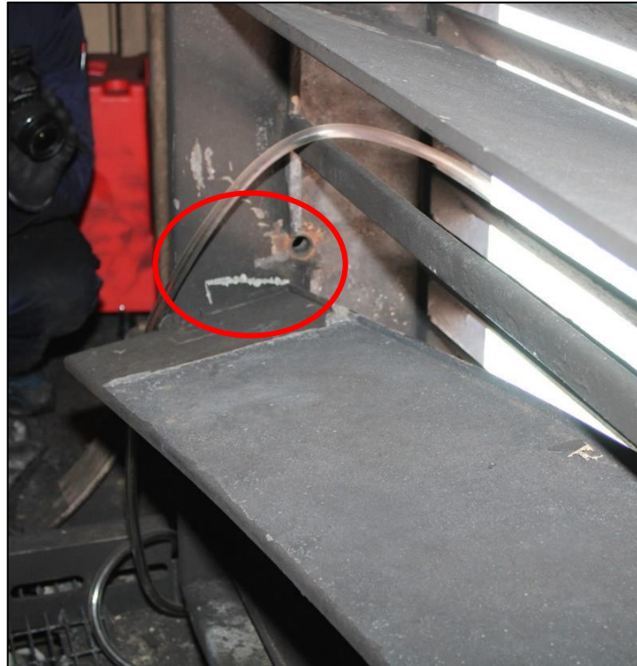
Figure 19: Lower louver seen in a clean state
