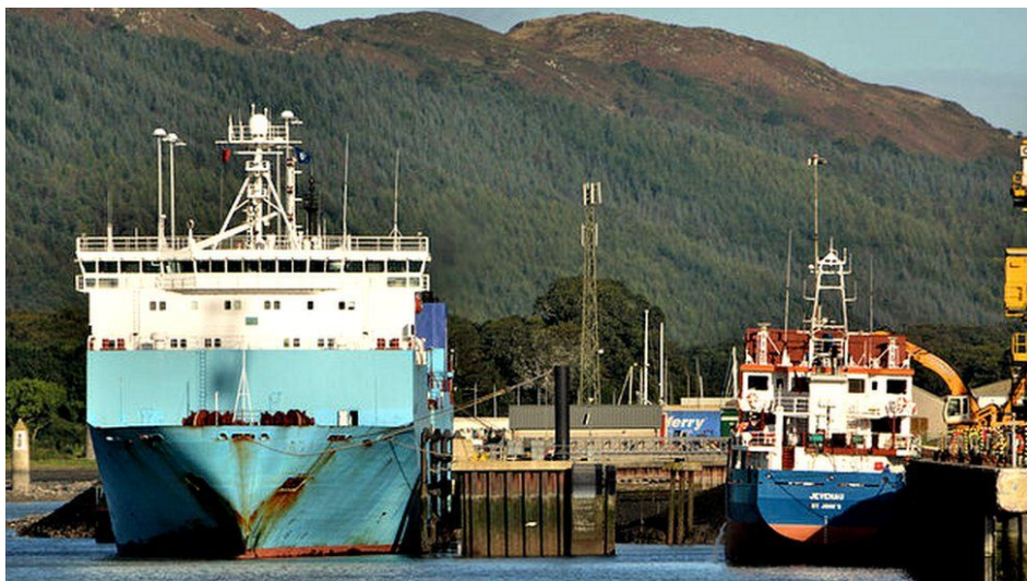
Figure 9.1 – Warrenpoint Harbour Facility [3]
