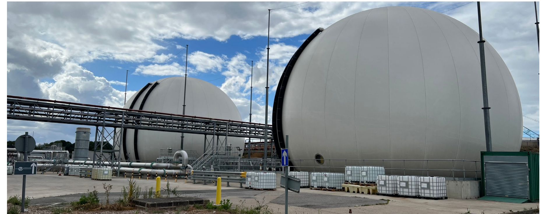
Bio-gas storage tanks in a wastewater treatment plant in Billingham, UK.
