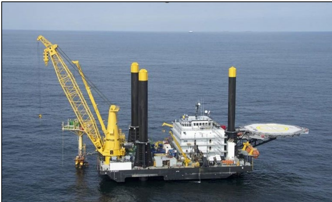
Figure 1. L/B Robert elevated and operating alongside a platform precasualty. (Source: Peter Dieter Janson)
