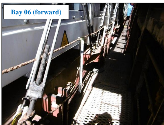
Figure 2: Stanchions and rope fitted on the forward side of bay 06
