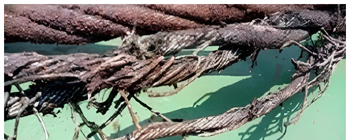
Parted crane wire
