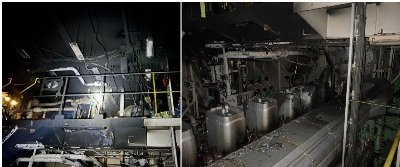
Figure 4. (Left) Smoke and fire damage to the upper engine room postcasualty. (Right) Fire origin and damage to the starboard engine and upper engine room postcasualty.
