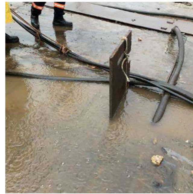
Drainage system unable to cope with the volume of rainwater at the time of the inspection.
