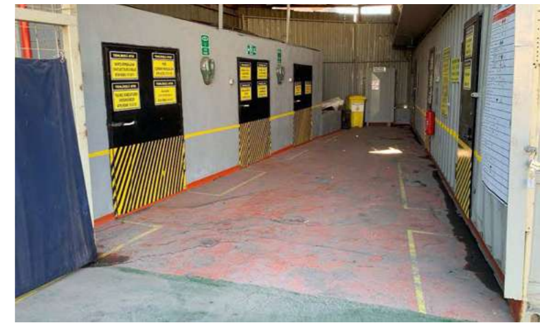
View inside the hazardous waste temporary storage area Source: Site Inspection Report of BMS (19.9.2022)
