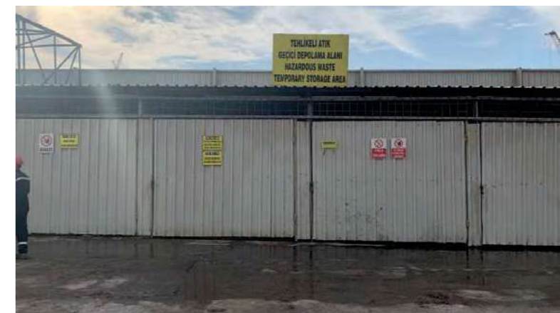
Temporary storage area for hazardous waste Source: Site Inspection Report of Kılıçlar (10.10.2022)
