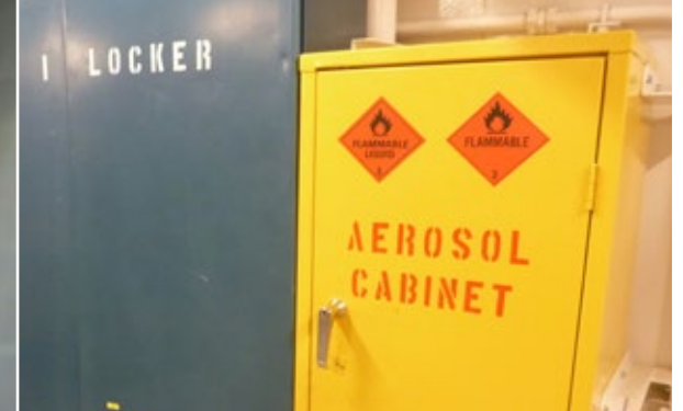
! Safe and secure stowage of paints and other flammables including safety data sheets (SDS), PPE (e.g. eye protection) and emergency eye wash bottles readily available. Fire protection in accordance with applicable regulation
