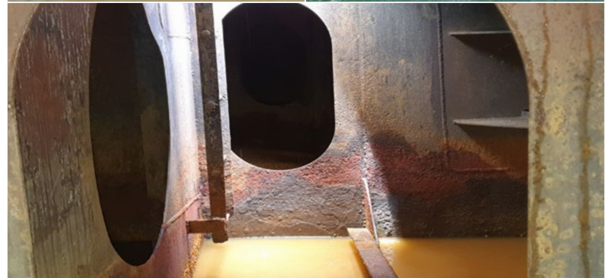
! Vessel and barge draught marks and water in void space.
