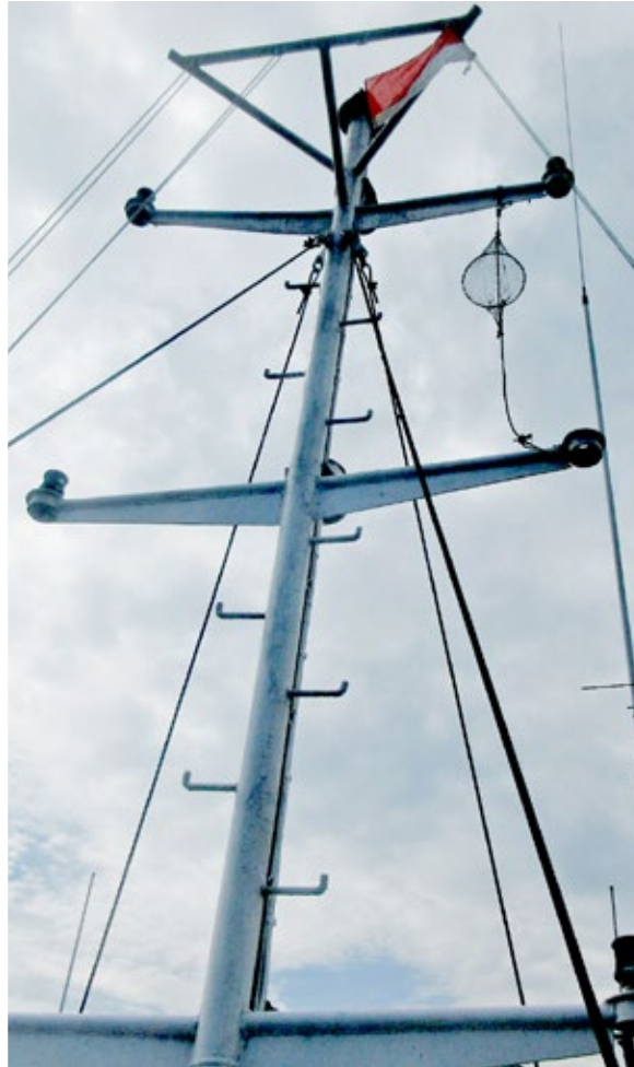
! Work at height could be prevented by using a halyard instead of fixing this day signal up the mast.
