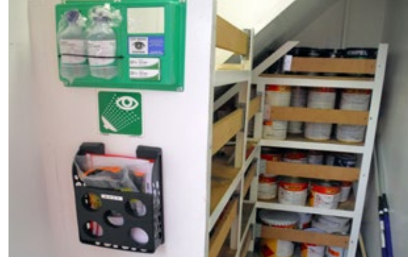
! Safe and secure stowage of paints and other flammables including safety data sheets (SDS), PPE (e.g. eye protection) and emergency eye wash bottles readily available. Fire protection in accordance with applicable regulation
