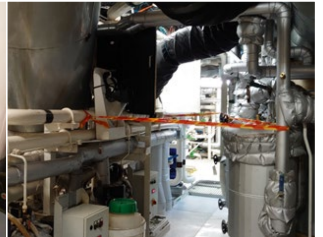
! Stanchions and chains/bars readily available at low level hatches, and tape used in other areas to control access
