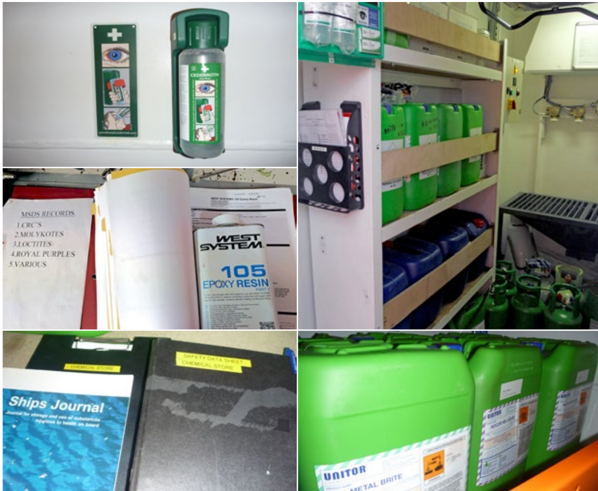
! Safe and secure stowage of chemicals, including safety data sheets (SDS), PPE (e.g. gauntlets, apron, face shield), and emergency eye wash bottles readily available. Containers properly labelled.
