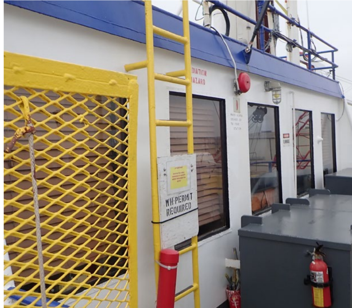
! Fixed ladder blocked with PTW signboard. Example PTW form. Active permits posted.
