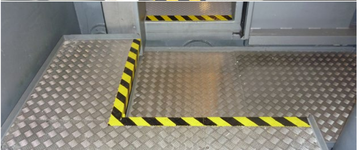
Safe walkways and good highlighting of changes in deck level and permanent trip hazards
