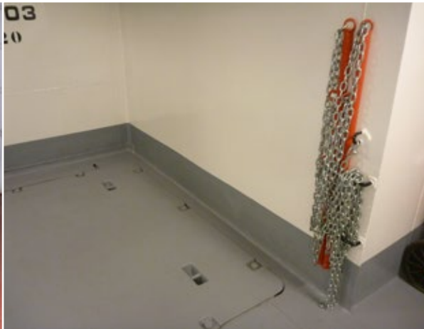
! Stanchions and chains/bars readily available at low level hatches, and tape used in other areas to control access
