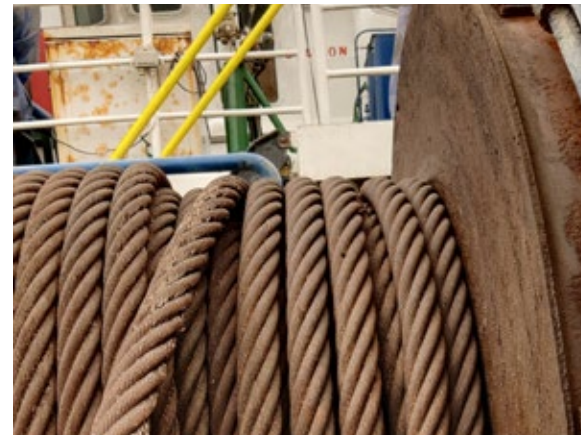
! Wire ropes should be routinely inspected and greased as applicable.
