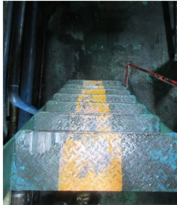
X Slip hazards. Oil is particularly hazardous as it is easily spread and is not always visible
