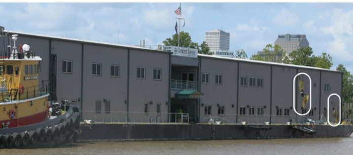
Figure 47. Office barge with detached mooring apparatus and structural penetrations (outlined in white).
