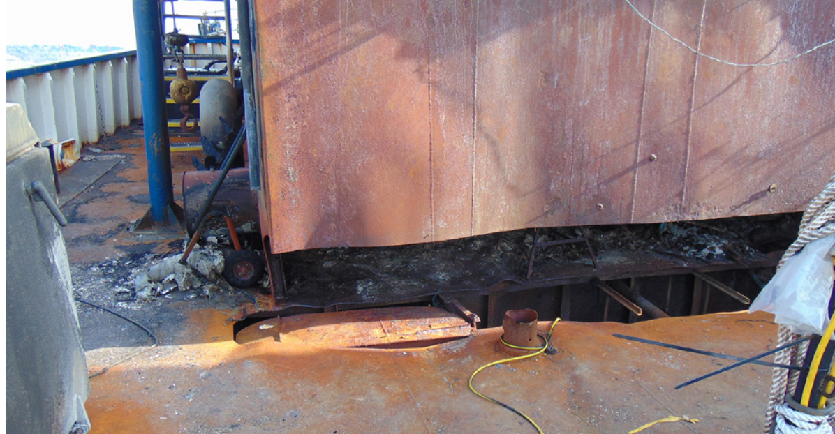
Figure 66. Aleutian Falcon bridge deck post-fire, depicting hot work area on the day of the casualty.
