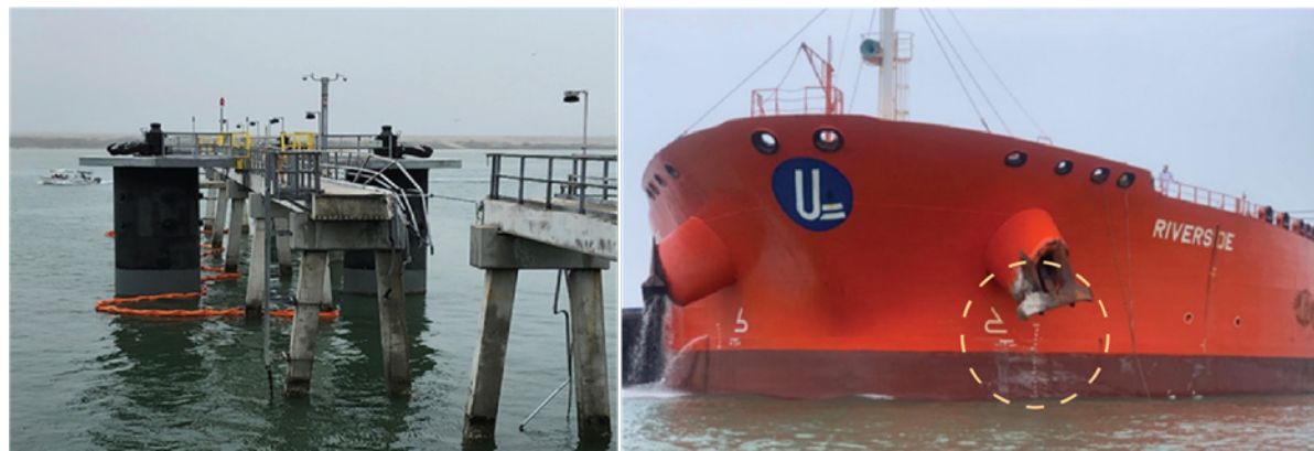
Figure 58. Damage to the no. 4 Moda dock catwalk (left) and the Riverside (right, circled). SOURCE: COAST GUARD
