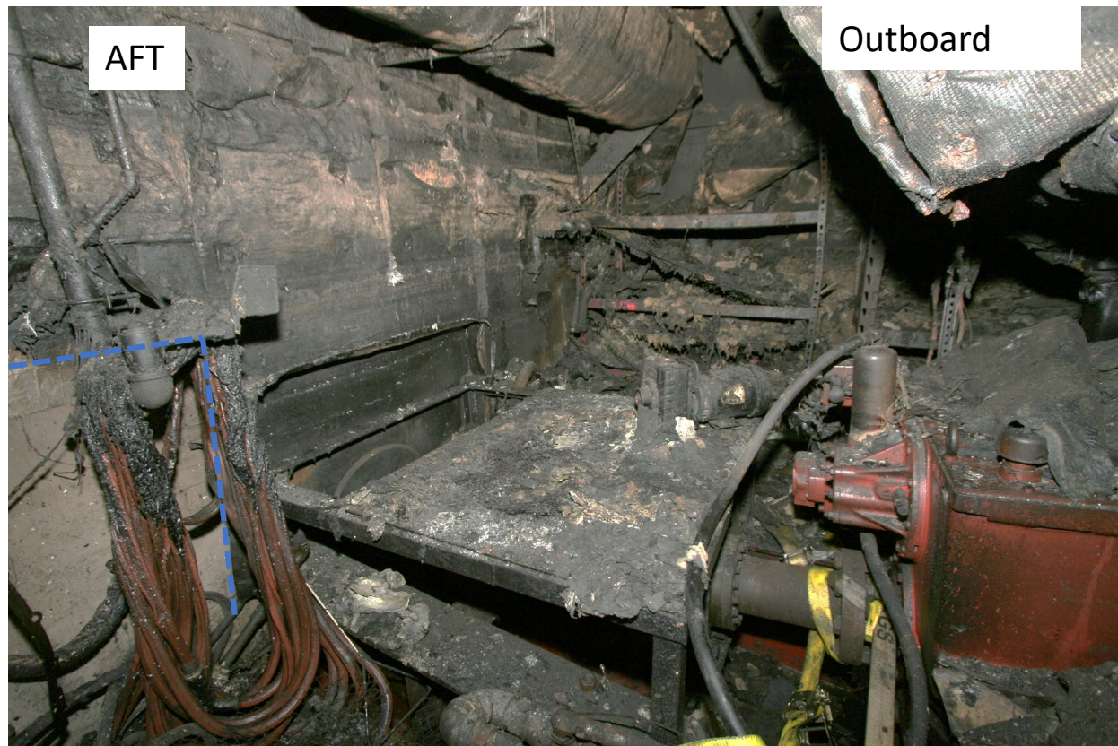
Figure 12. Fire damage on the bulkhead aft and outboard of port main engine. The metal frames of the storage shelves are visible against the bulkhead.
