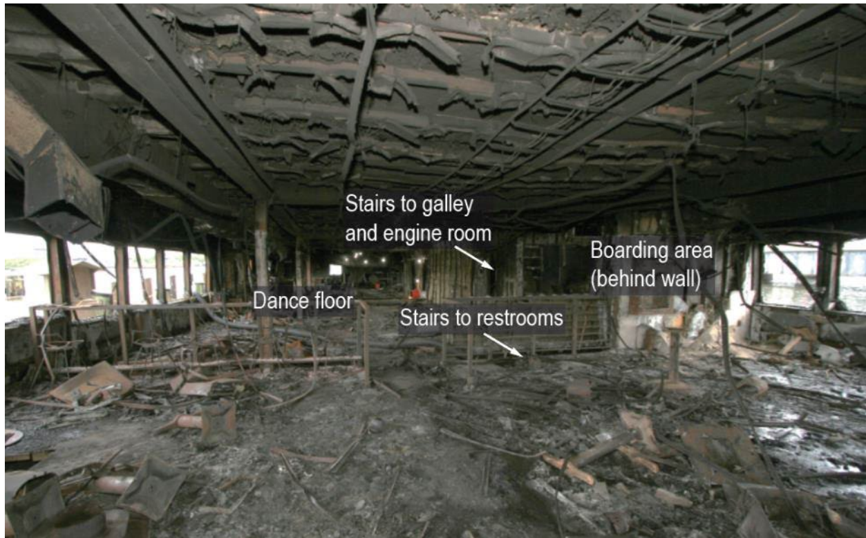
Figure 14. Main deck interior looking aft.
