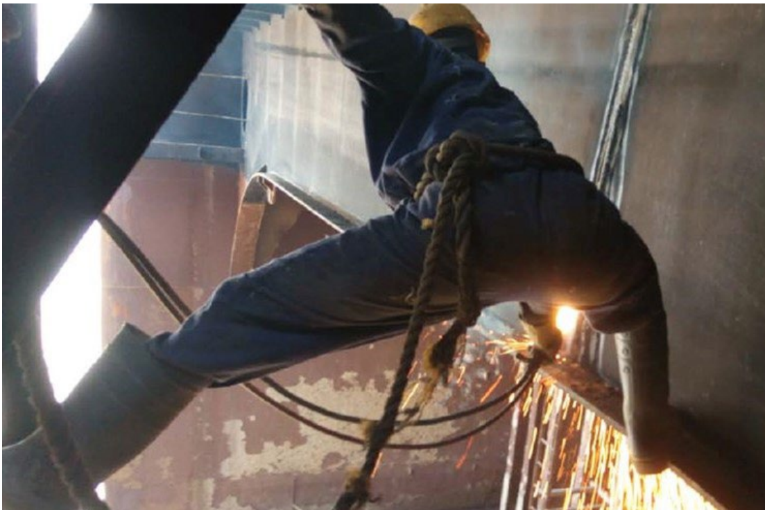
A shipbreaking worker balances on the ledge of a ship to torch through the steel. © 2023 Anukta
