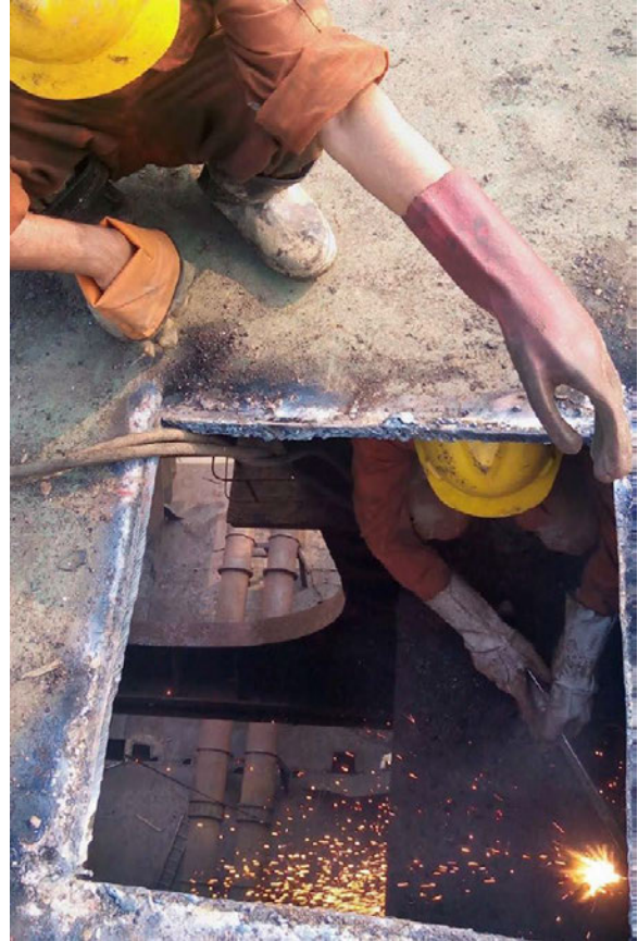
Shipbreaking workers cut through steel inside a confined space. © 2023 Anukta
