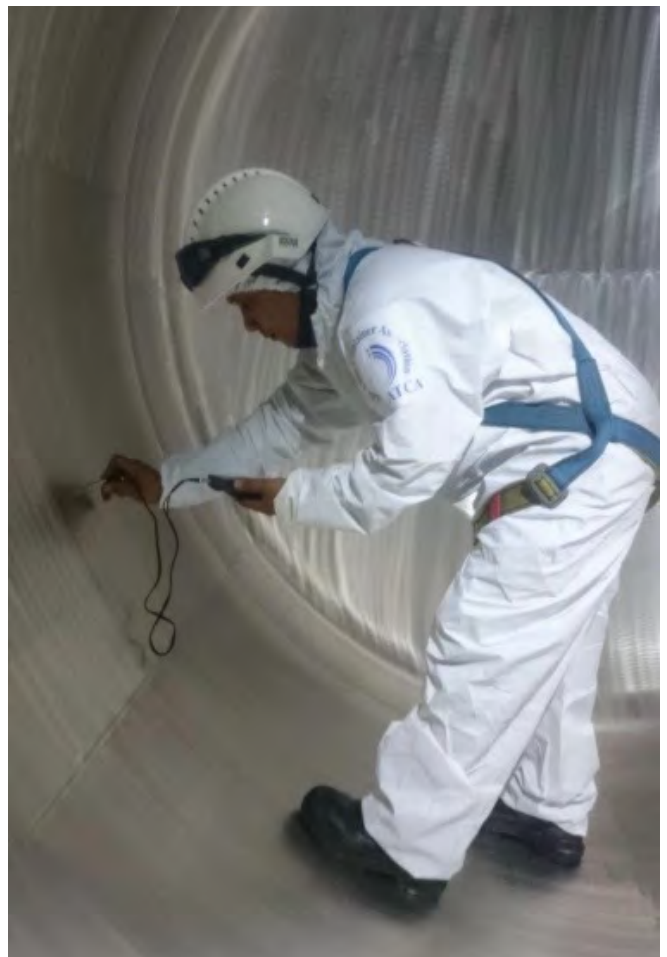
Inspector measuring the shell thickness from inside the tank.
