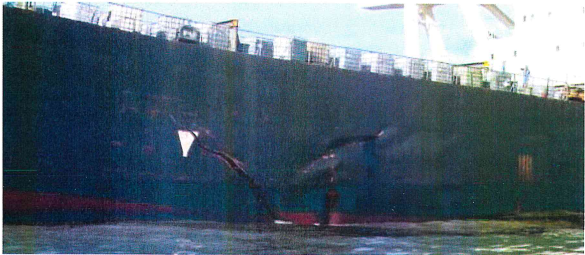
Figure 7, PS crack at Frame 91.
