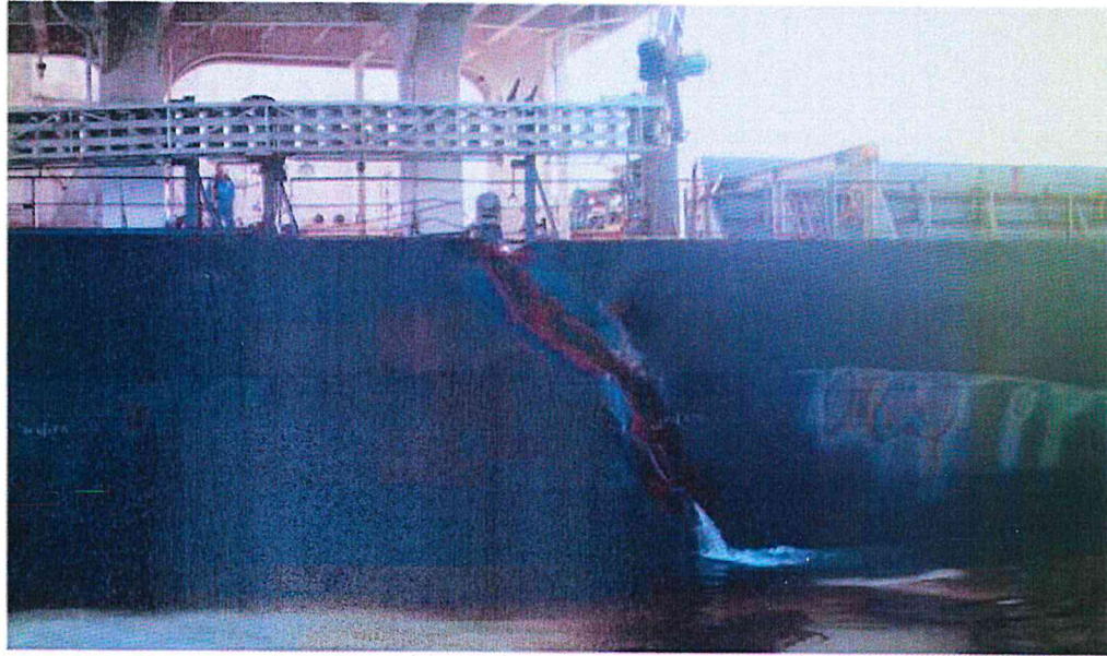
Figure 11, SB crack at frame 42
