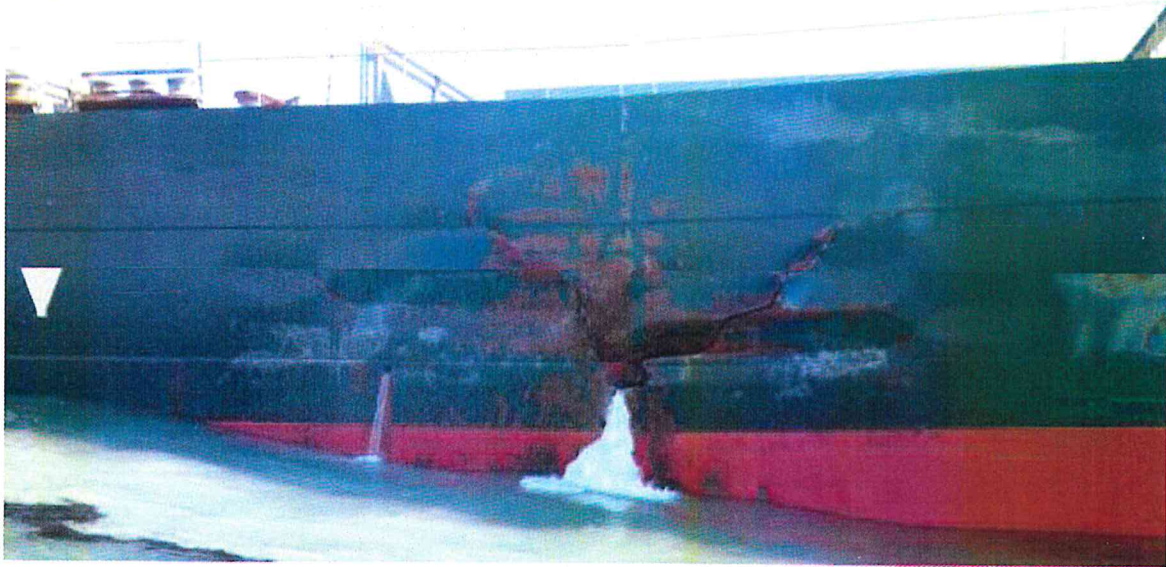
Figure 3, SB crack at Frame 83
