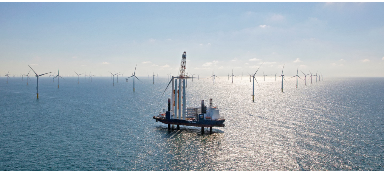
Figure 9: Offshore wind installation vessel. Image reproduced with permission from Van Oord.
