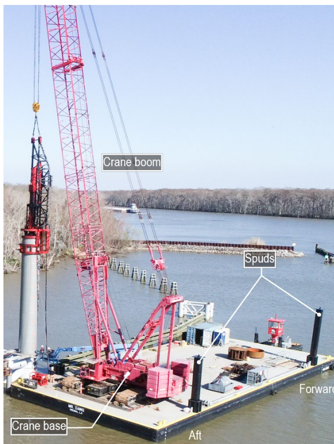
Figure 3. Crane barge Mr. Dawg in operation. (Source: Houma Times)
