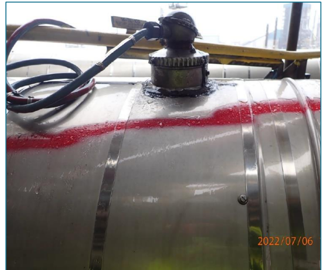
Figure 10 Photographs showing that thermowells on pipes between reactors and heaters with and without insulated flanges. Photos: Equinor
