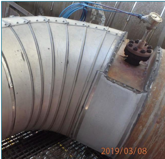
Figure 10 Photographs showing that thermowells on pipes between reactors and heaters with and without insulated flanges. Photos: Equinor
