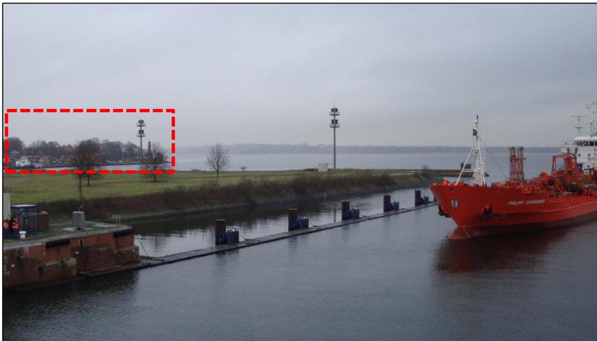
Figure 36: View from the lock control station in Kiel-Holtenau towards Kiel Fjord
