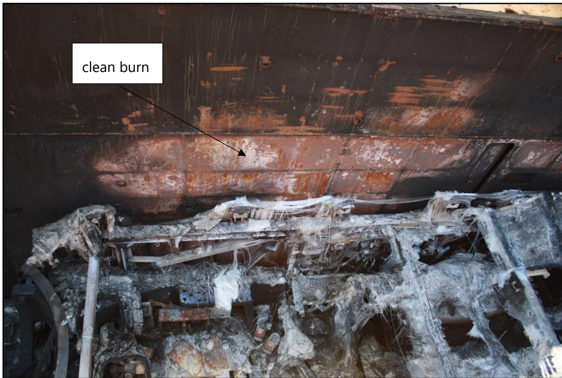
Figure 14: Fire-damaged nacelle and clean burn pattern, port side aft number 2 'tween deck
