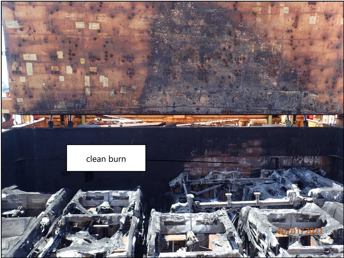
Figure 13: Number 2 cargo hold looking aft
