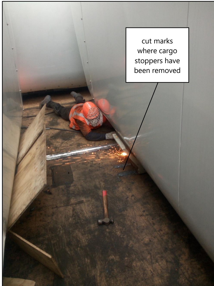
Figure 6: Gas-cutting removal of cargo stoppers (Credit: Used with photographer's permission)
