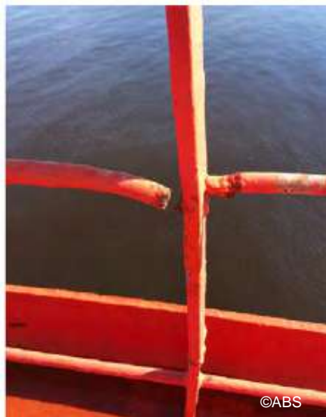
Load Line rail broken
