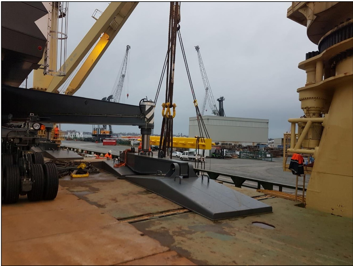
Figure 18: Crane 2 with double supporting pad (photograph taken after loading)
