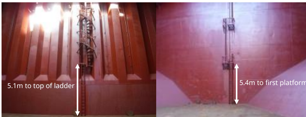
Spiral and vertical ladders in hold 7
