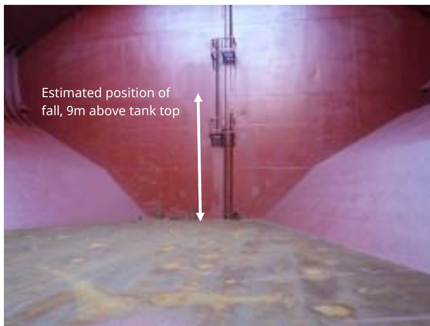
Hold 7: vertical (aft) ladder
