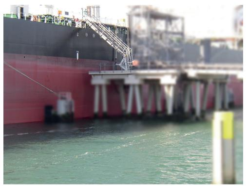
Figure 4: Gangway not suitable for operational envelope
