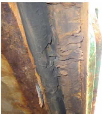
Figure 5: Hardened indented rubber seals
