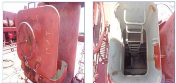
Figure 2: Access trunk hatchway and vertical ladder leading to pipe tunnel
