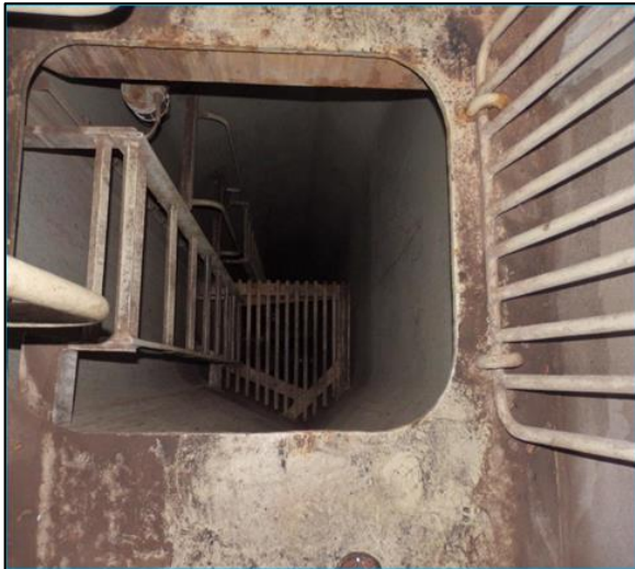
Figure 4: Photo showing platform A and vertical ladder leading to platform B
