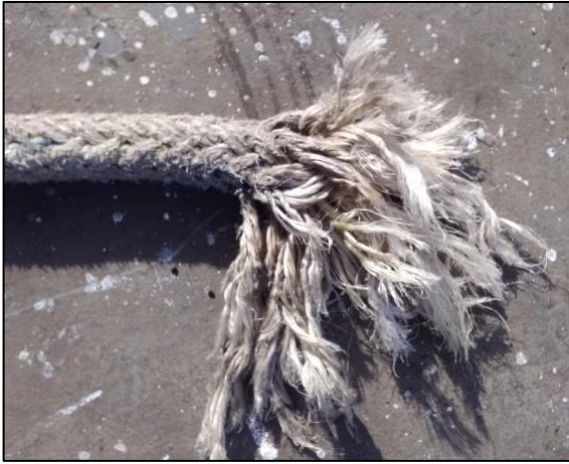
Figure 12: A section of the failed mooring rope
