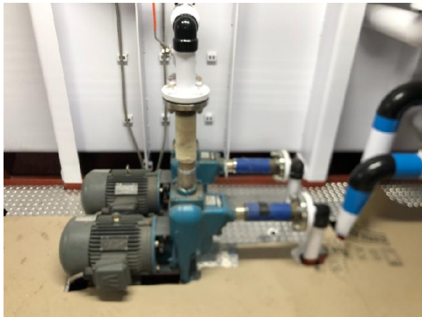
A typical dewatering pump arrangement for a towing vessel.
