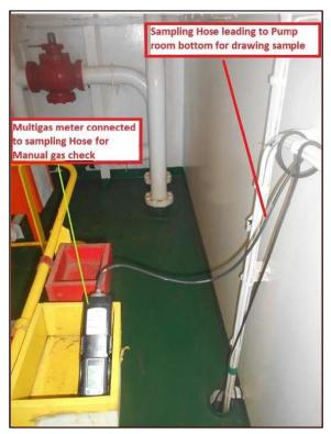
Figure 12: Personal multi gas detector placed at the pump room's entrance
