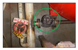
Figure 15: Suction valve (circled in green) of the starboard bilge of the pump room
