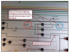
Figure 16: Location of the pump room's starboard bilge suction valve (circled in blue)
