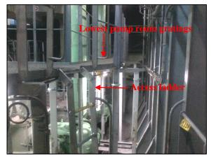
Figure 5: Access towards starboard side bilge alarm sensor
