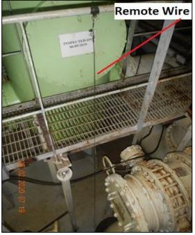
Figure 17: Wire to remotely test the starboard bilge alarm
