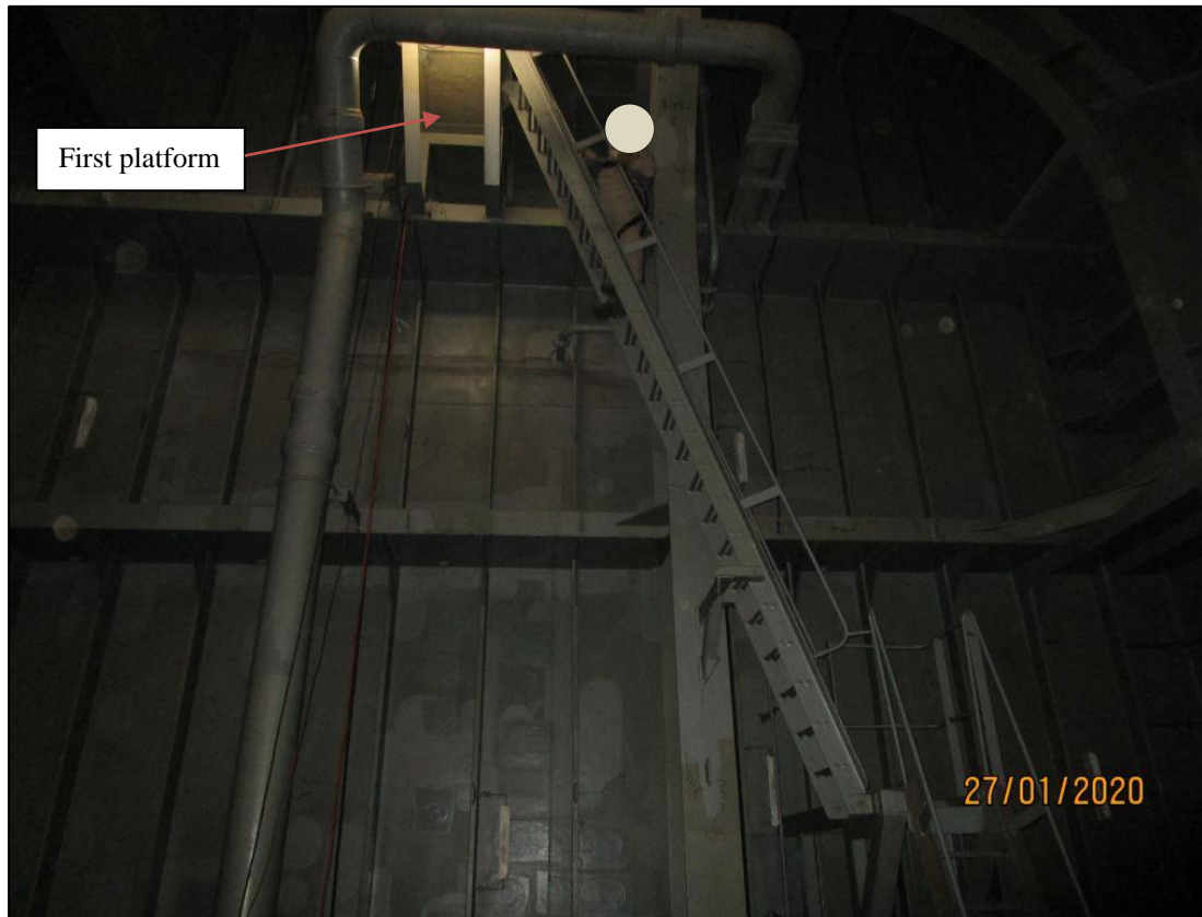
Figure 9: Access ladder inside water WBT no. 1006
