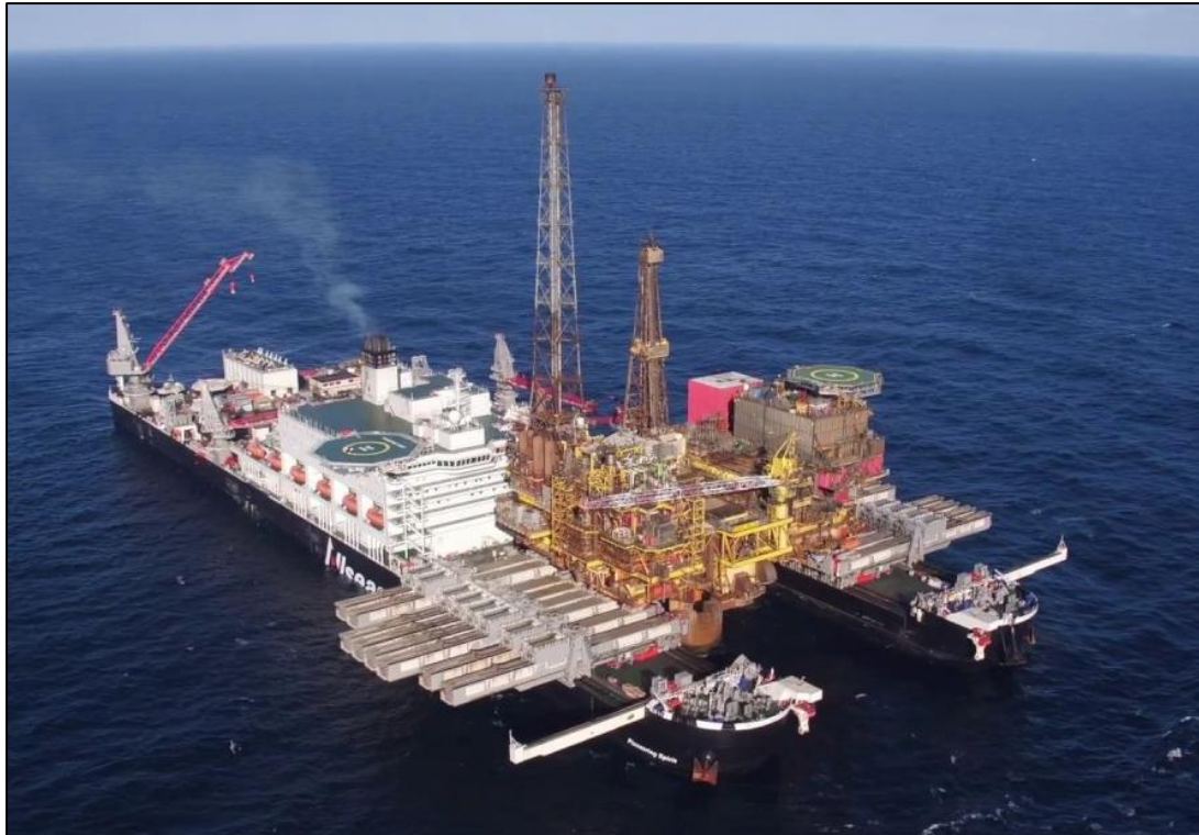
Figure 2: Pioneering Spirit carrying topside
