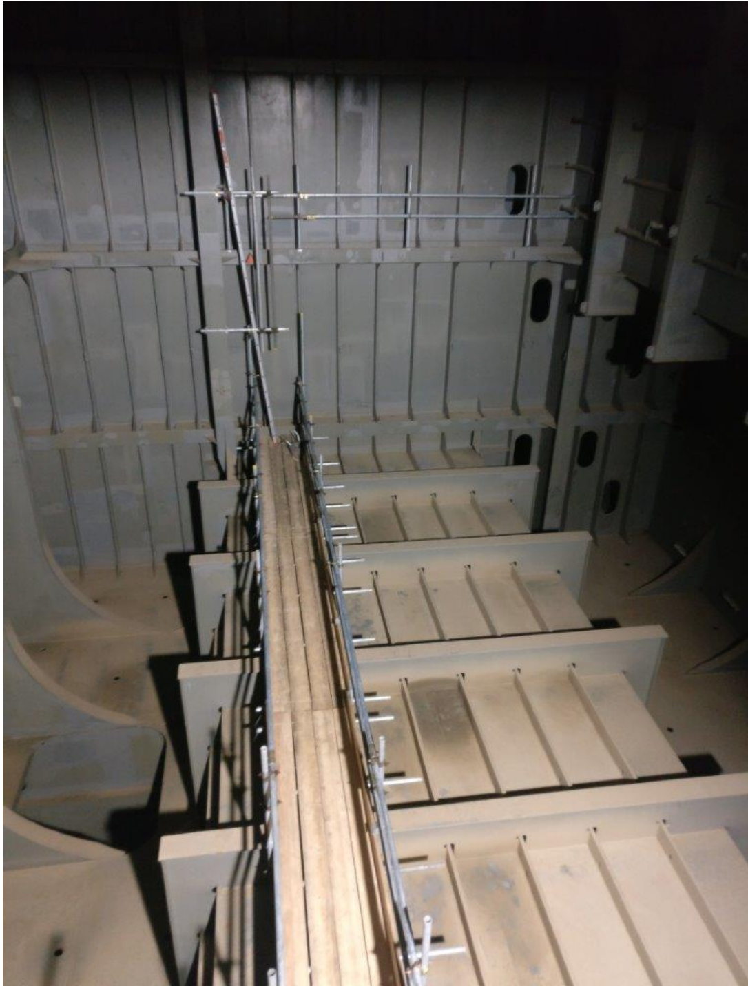
Figure 13: Scaffolding during initial work in tank in October 2018
