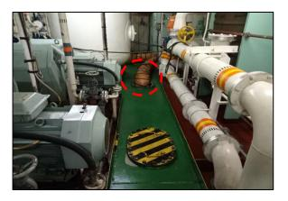
Figure 4: Access manhole of the grey water tank with the ventilation duct in place
