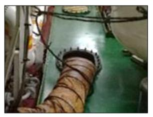
Figure 9: Ventilation duct passing through the grey water tank manhole
