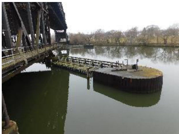
Left: Northeast protection cell for Rock Island Railroad Bridge. Right: View from across the river of damaged protection cell with impact location circled. (Source: CSX Transportation)
