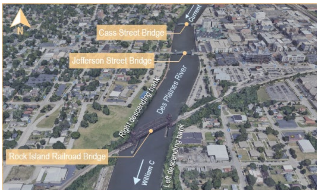
Bridges through which the William C 's tow transited. (Background source: Google Earth)
