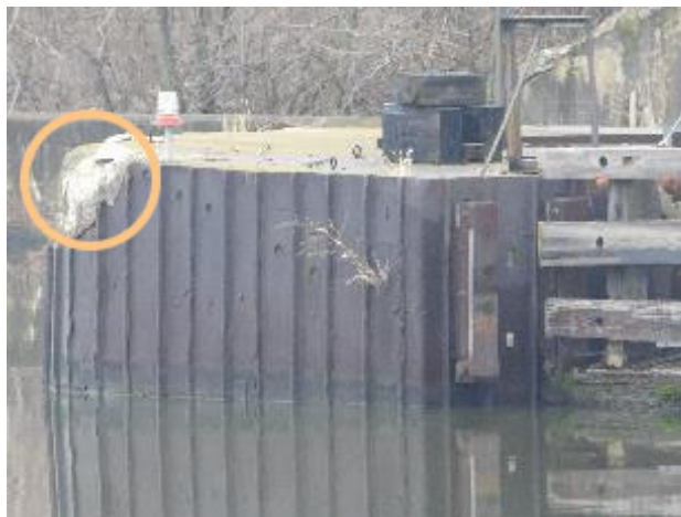
Left: Northeast protection cell for Rock Island Railroad Bridge. Right: View from across the river of damaged protection cell with impact location circled. (Source: CSX Transportation)
