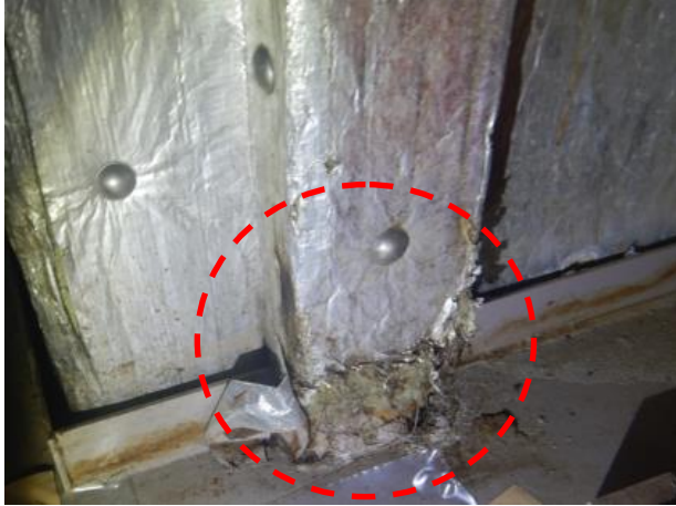
← Deteriorated insulation
