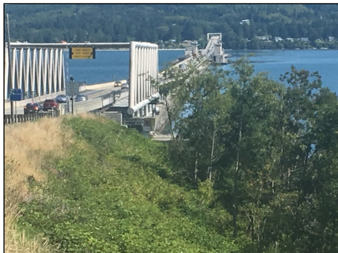
Hood Canal Bridge from Termination Point looking northeast. The east span is shown on the left.
