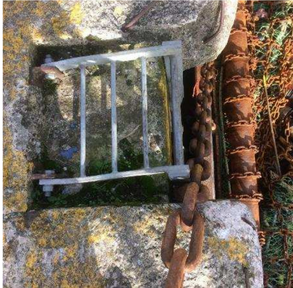
Figure 5 - Quay side ladder- top view from jetty
