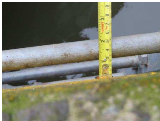
Figure 13 - Quay side ladder detail - Distance between concrete and supports
