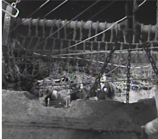
Figure 9 - Chains of fishing gear obstructing quay side ladder (1)
