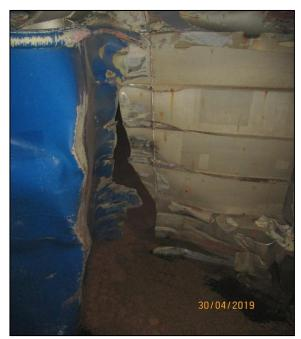
Figure 7: Structural damages in way of the cargo hold
