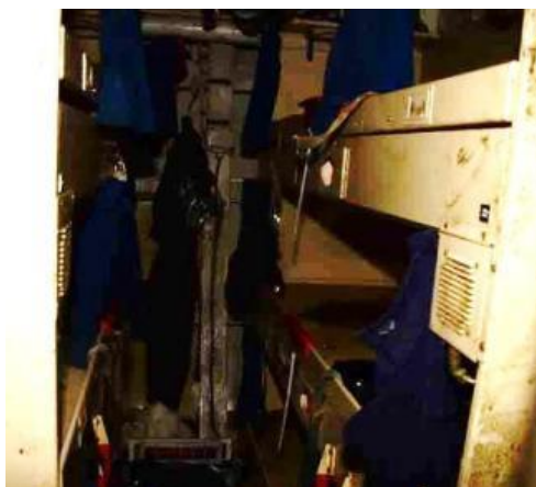
Figure 18—Berthing 4 racks after dewatering
