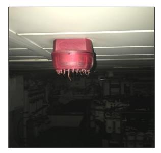
Figure 9: Heat detector, located above the port side engine
