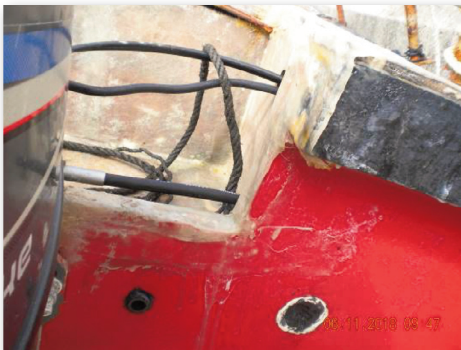
Photograph No. 4: Hole is in starboard side of transom, one for steering cable and the other for original exhaust outlet.
