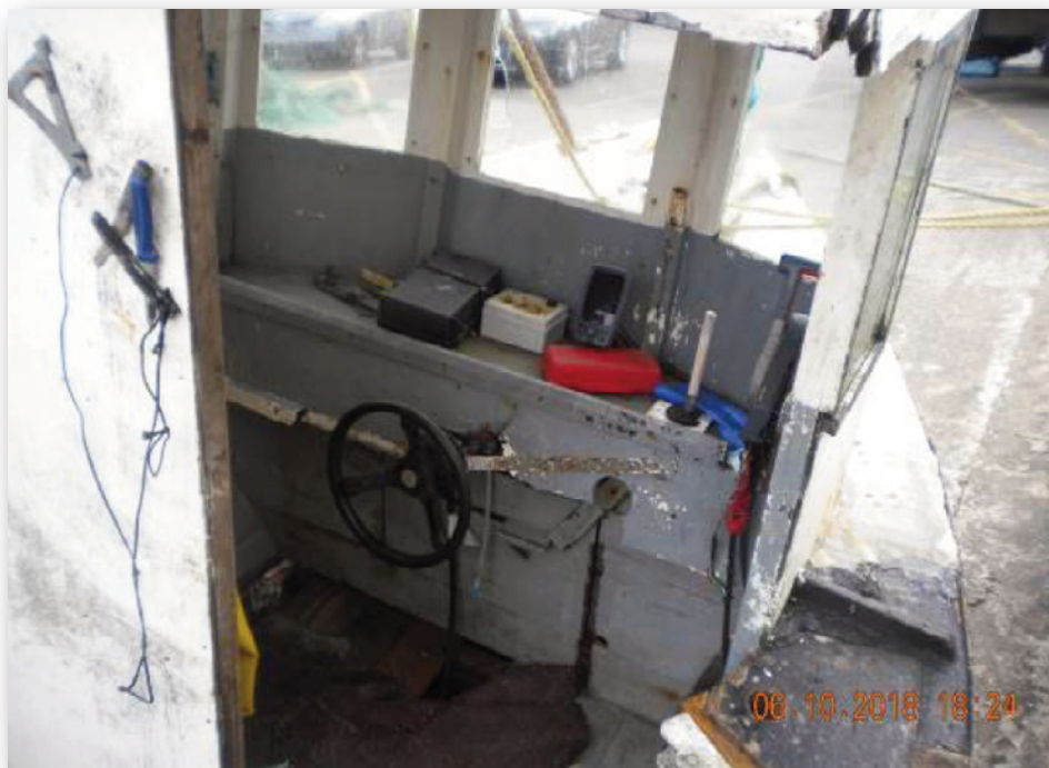
Photograph No.3: View of wheelhouse interior.
